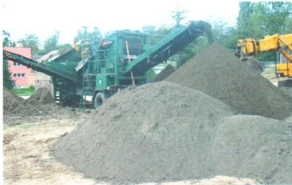
Building waste recycling screen undersizes fraction
